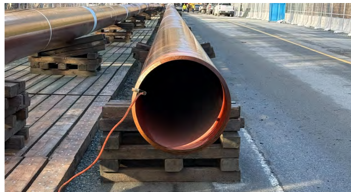
24' pipe to be installed
