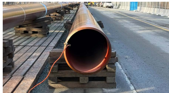
24' pipe to be installed
