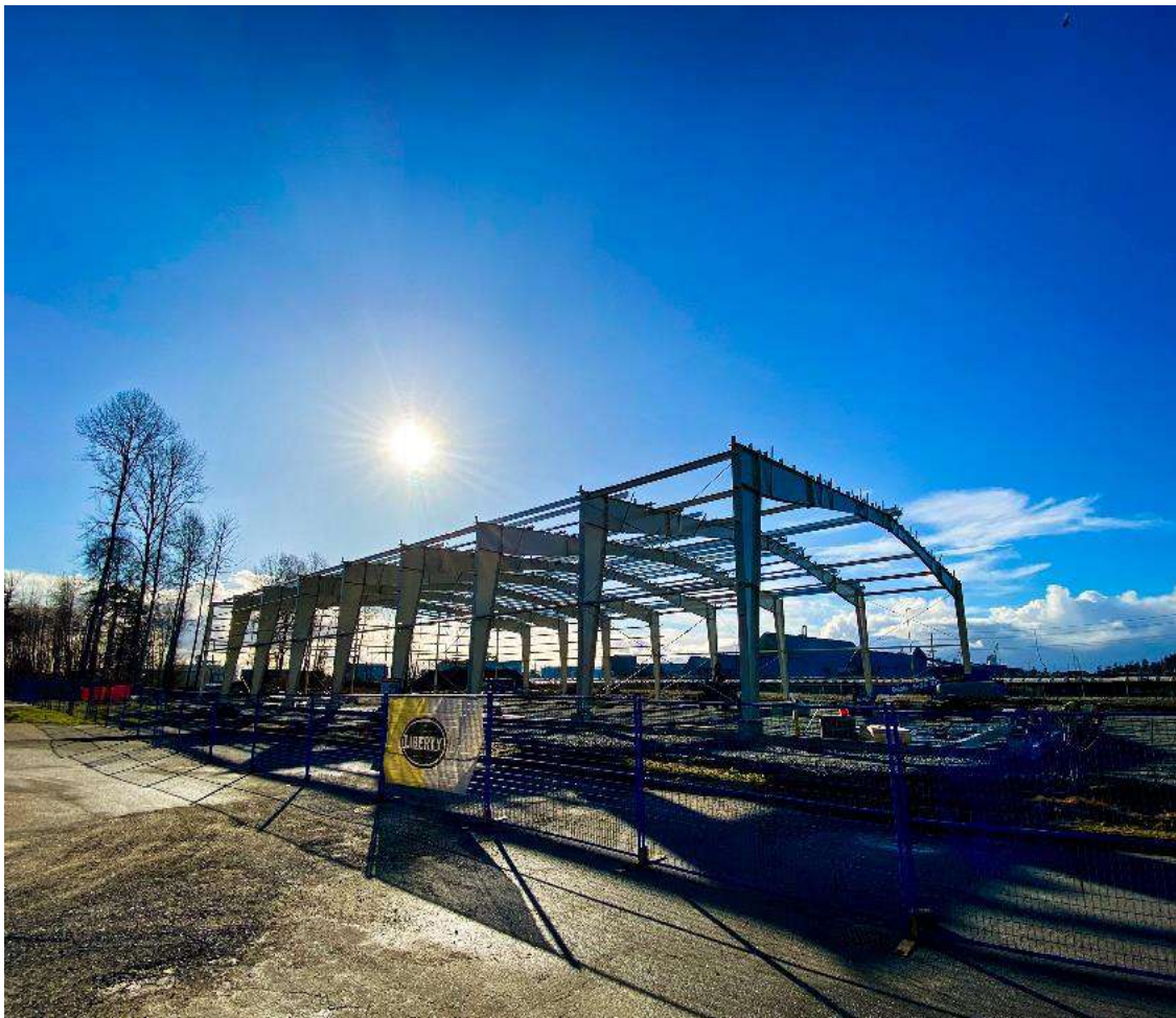
Figure 1. Roof Structure Construction (March 23, 2024)
