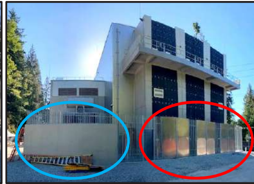
North-west corner of substation (blue) and six aluminum panels for optional wraps (red)
