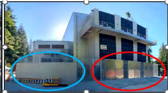
North-west corner of substation (blue) and six aluminum panels for optional wraps (red)
