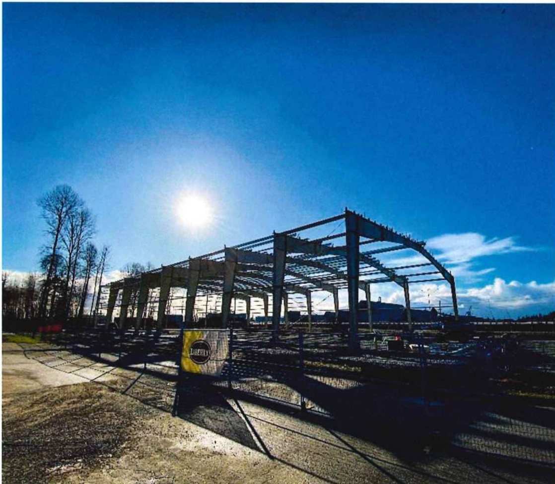
Figure 1. Roof Structure Construction (March 23, 2024)
