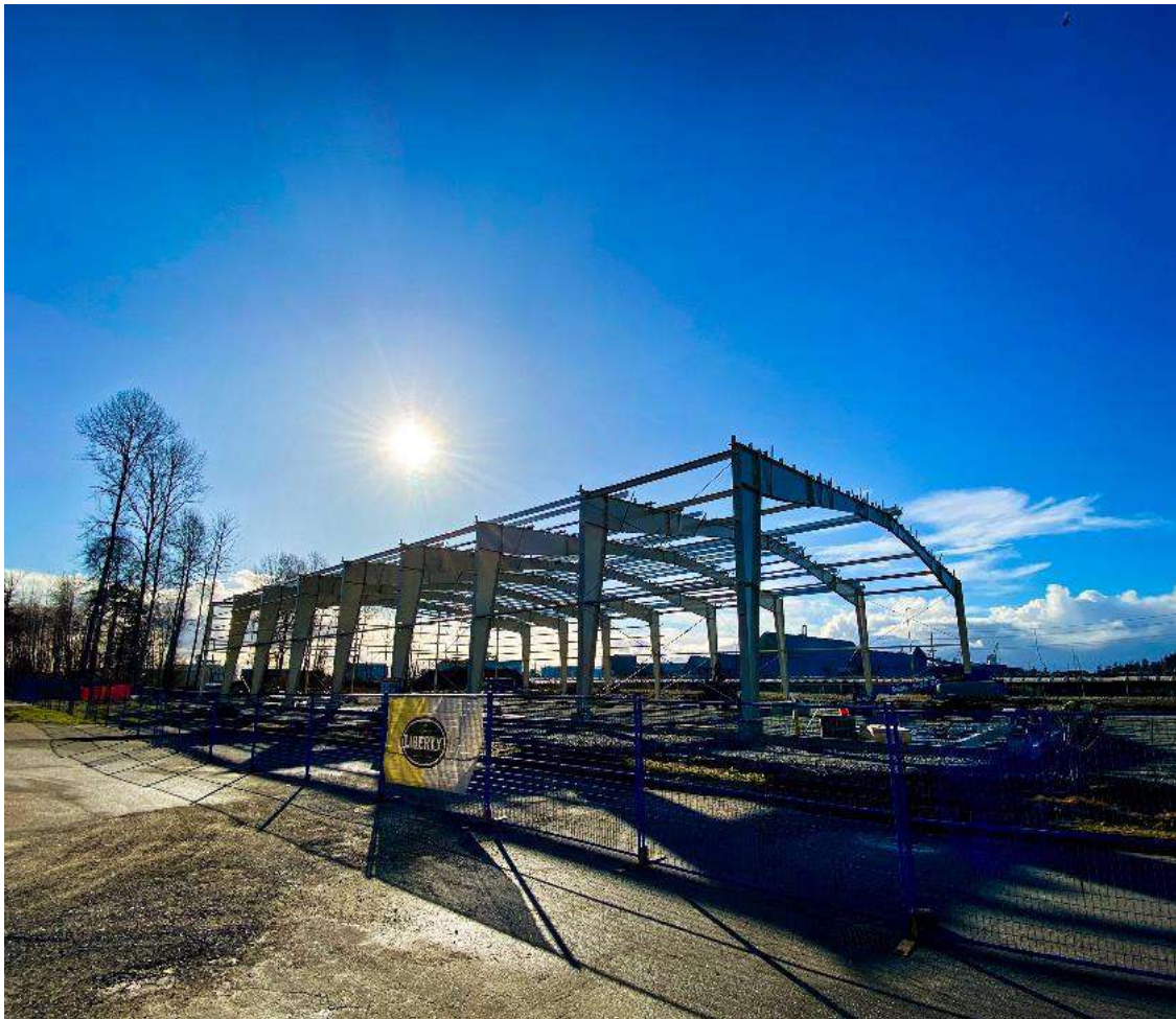
Figure 1. Roof Structure Construction (March 23, 2024)
