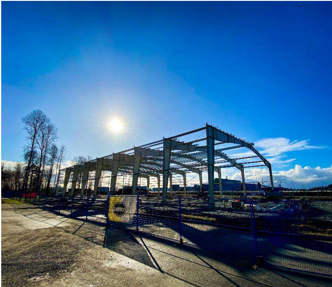
Figure 1. Roof Structure Construction (March 23, 2024)
