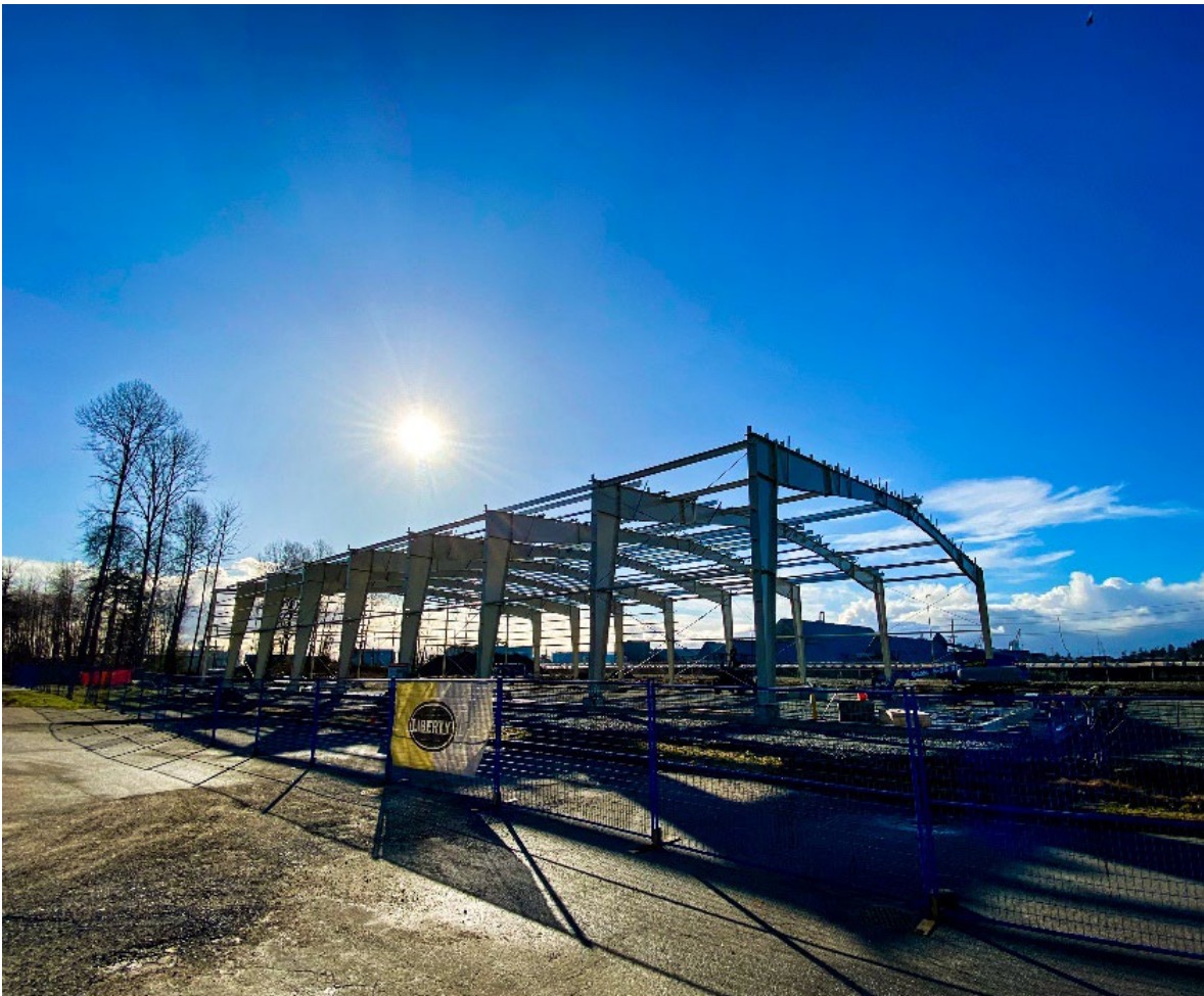
Figure 1. Roof Structure Construction (March 23, 2024)
