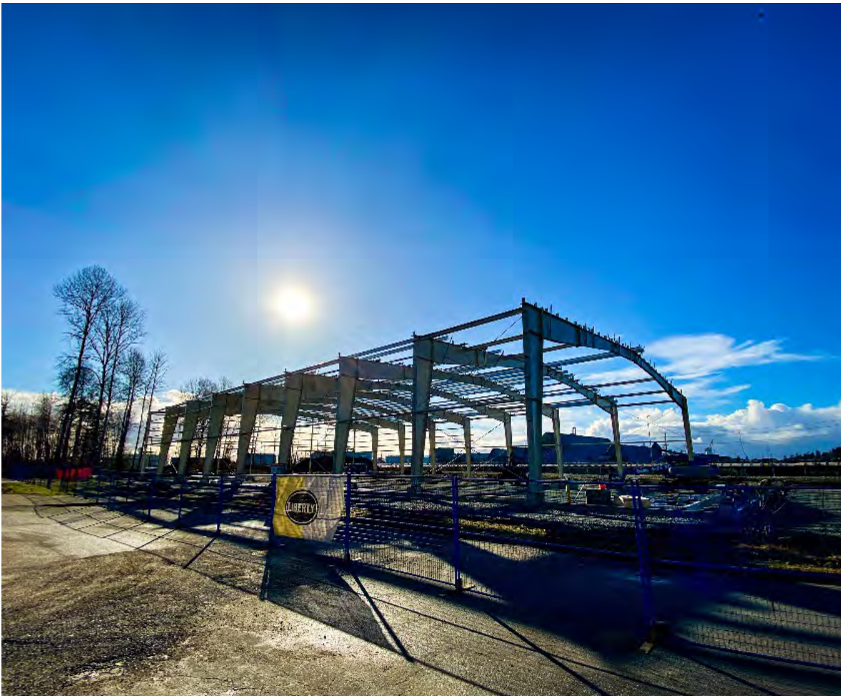
Figure 1. Roof Structure Construction (March 23, 2024)
