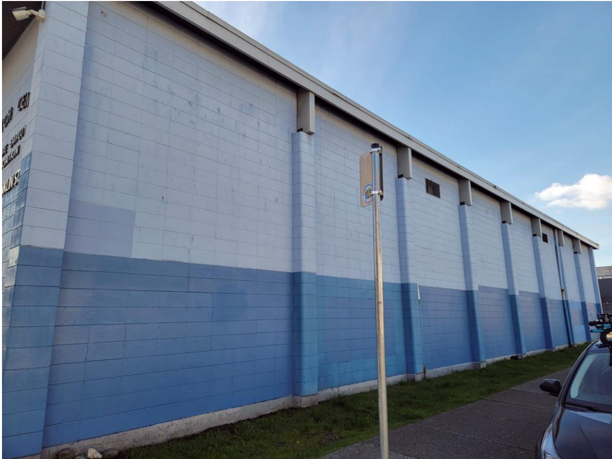
Figure 2. Photo of the North Elevation side wall of Dispatch Centre building
