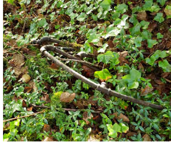
Floatel walkway route has lots of abandoned water pipes and heating tanks from when mill houses were located there in the 1960s.
