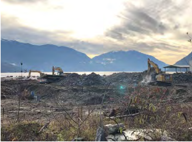
Concrete slab removal
