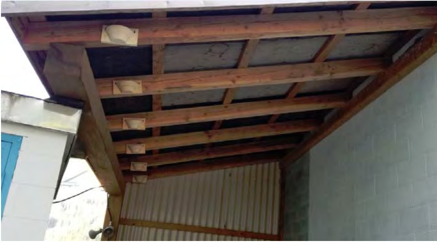
At the Woodfibre LNG site, new nesting cups for Barn Swallows are being used to replace nesting habitat removed when old buildings are demolished.
