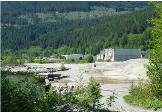
Woodfibre LNG site on 22 May 2019. Many of the old pulp & paper mill buildings and broken piers have been removed.
