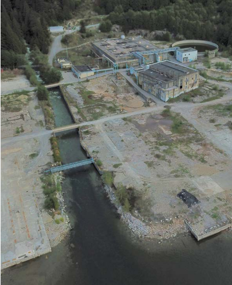
Mill Creek –previous site development left minimal riparian (streamside) vegetation and concrete walls instead of banks, but it still supports salmon spawning
