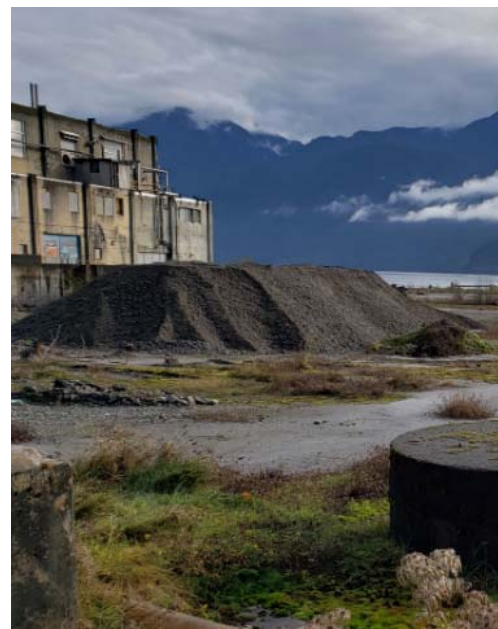
Site cleanup, November 2019
