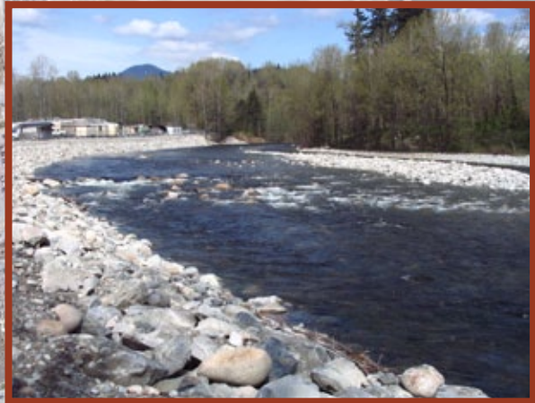
Seymour River Bank Protection
