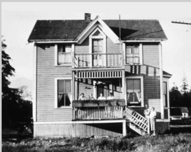
Newman house on Squamish Indian Reserve, foot of Capilano Rd. at First Narrows, circa 1930's. Source: Museum of North Vancouver Archives
